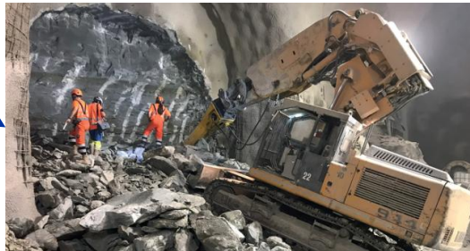
New service tunnels for the high-luminosity LHC being excavated at Point 5 in July 2019. Credit: Z. Arenas
