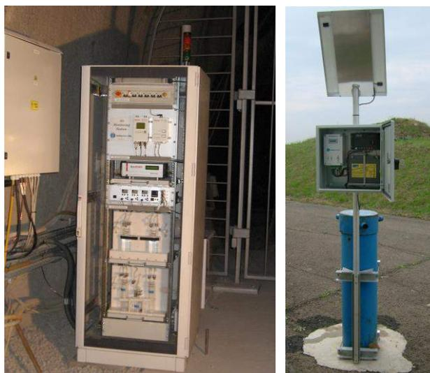
**Figure 61:** Air monitoring station installed in Bataapati and water monitoring station in Puspokszilagyi.
